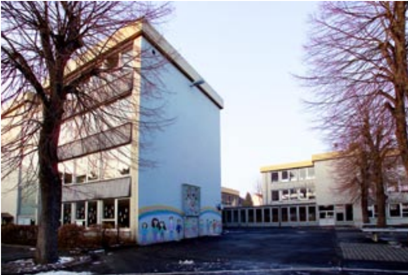
Geschwister-Scholl-Schule in Mühlheim am Main
